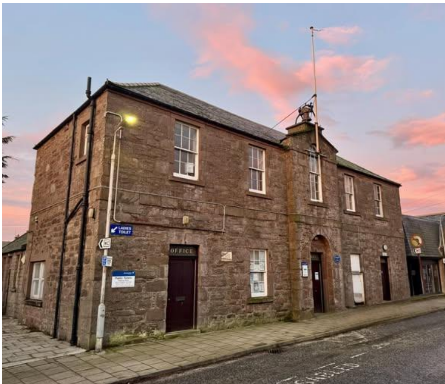
The Burgh Chambers building hosting the library and public toilets.
